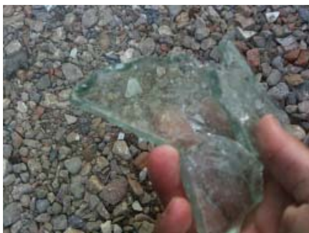
Glass in the hardcore at Alderley before the topping was added
